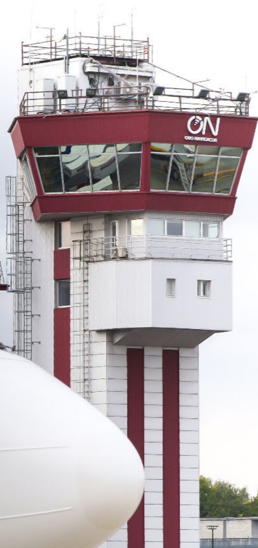
BELOW: The control tower at Vilnius airport ORO NAVIGACIJA
