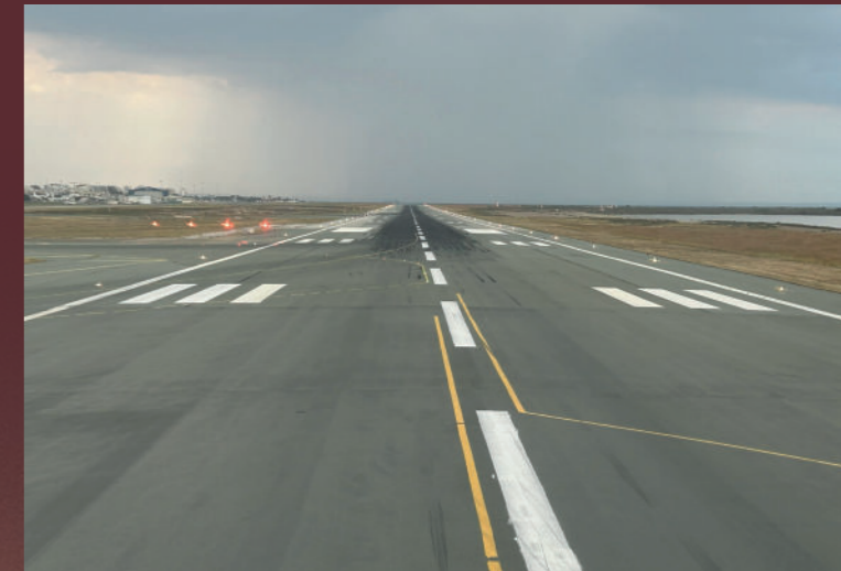
ABOVE: Lined-up on the runway at Larnaca airport
